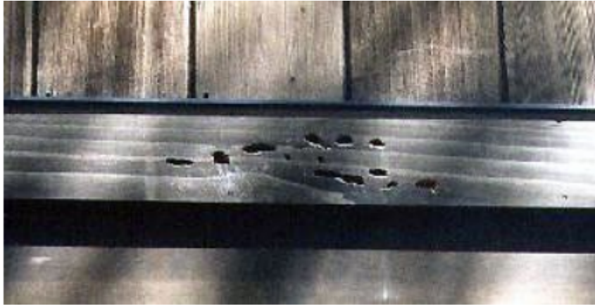
Woodpecker damage due to foraging for carpenter bee larva on cedar trim boards of a house.
